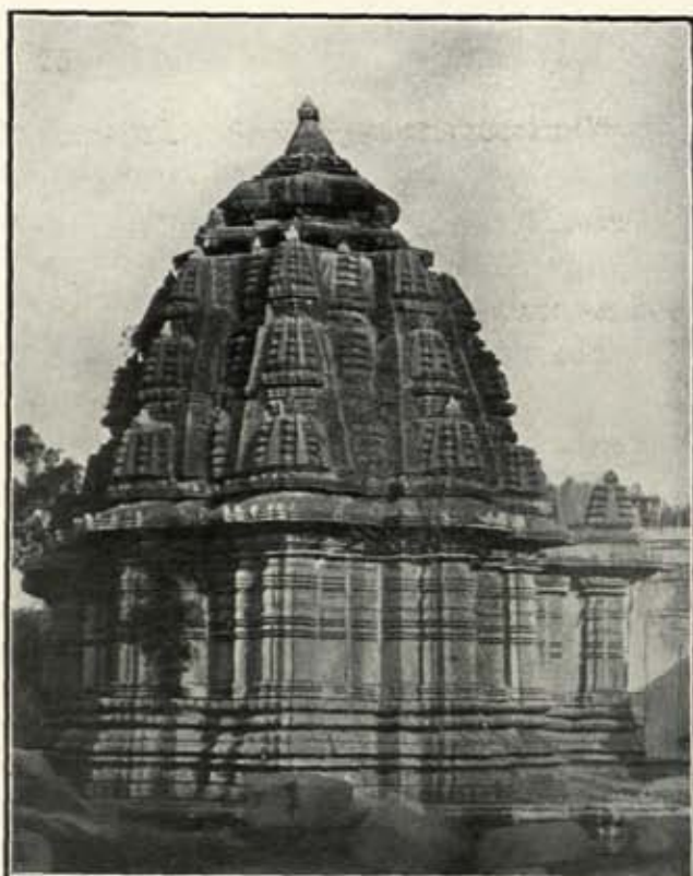
2. NUGGIHALLI: SADASIWA TEMPLE, SOUTH VIEW OF TOWER (p. 32).
